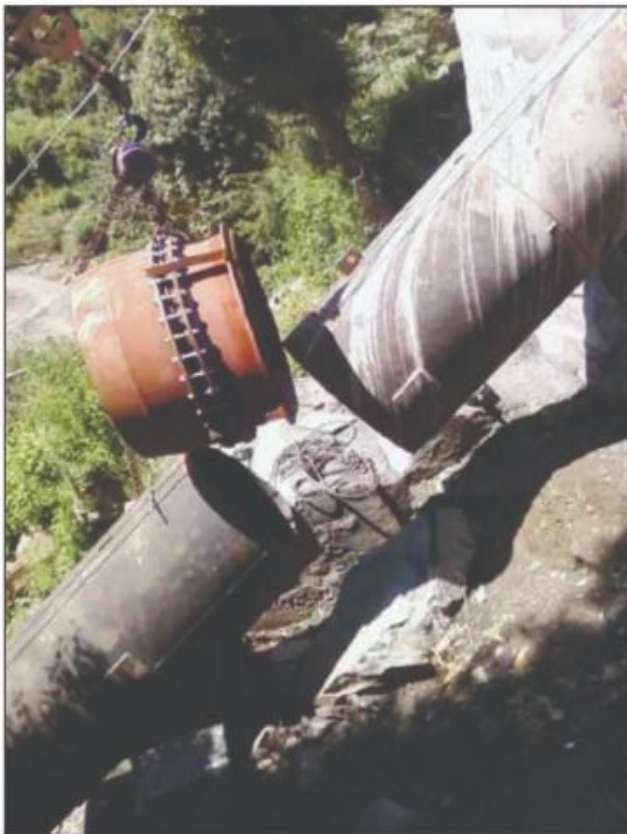
Expansion Joint being placed in position
