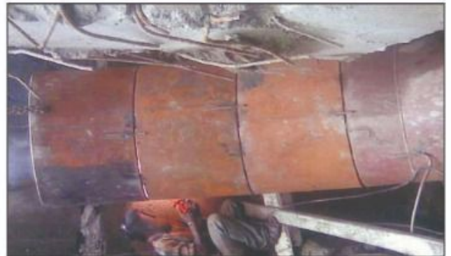
Bend fit-up in progress
