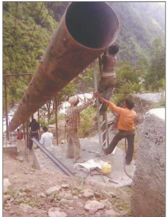
Penstock Erection in progress
