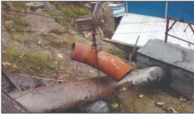
Reducing Bend being placed in position
