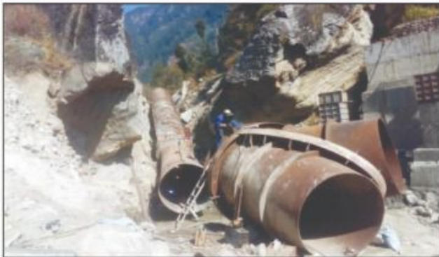
Bifurcation Pipe being welded at site
